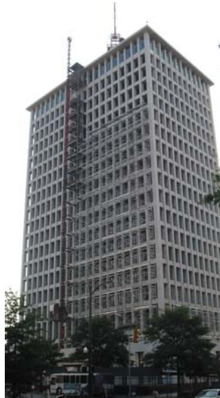
City Hall - Before
