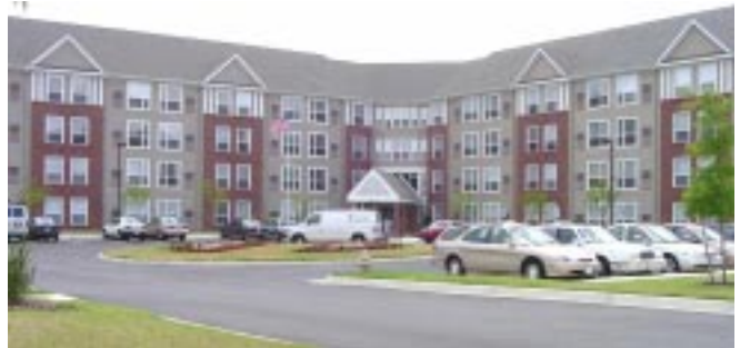
New construction at the Guardian Place Senior Housing Complex, north of Broad Street near I-195, added over 200 residents to the neighborhood.
